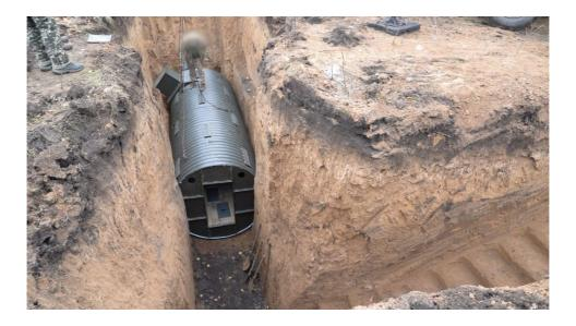
The next step involved much larger metal structures for shelter. Metinvest developed and launched the production of underground command posts designed for dozens of people from the Ukrainian armed forces command on the front line. Essentially, these are steel headquarters, a structure of five or six separate mobile bunkers, each of which has a functional purpose: living quarters, command headquarters, sanitary facilities and so on.
