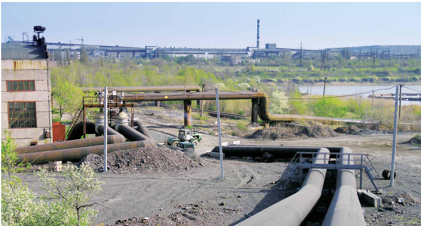
Construction of two gravity water conduits to supply process water to the ore preparation plant in Ingulets GOK
